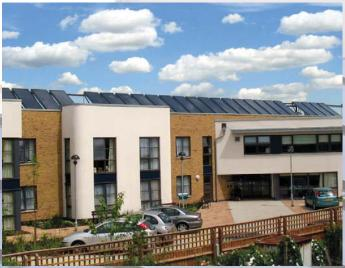
Extracare units, hotels, sports and medical buildings generally have a centralised plant room, so a solar heating system can pre-heat water in large buffer vessels.
