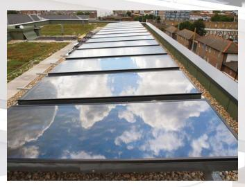
Panels can be installed on flat roofs at different pitch angles to optimise energy yield per unit area of roof, energy yield per solar panel, or to take account of planning restrictions on the height of the roof. Is solar heating an option?
