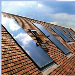
Clearline solar panels are lighter than the tiles they replace, removing the need for structural work in retrofit situations.
